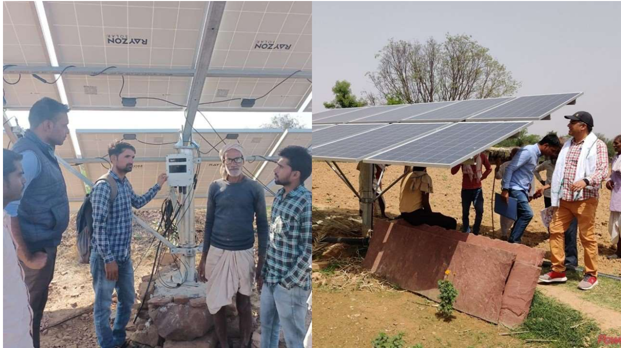
Installation of Solar Irrigation Pumps at Farmer's Field
