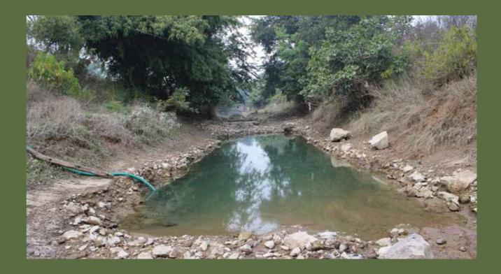
along with providing for excavators. The community was responsible for doha excavation operations, contribution of labour for transport and application of silt on farms and bunding of the Dohas. 23 Doha structures, measuring 20x5x1.5 mt (length x breadth x depth), were dug along a 3-kilometre stretch of the Bargi nala, flowing between Dor and Kharoi villages. The silt excavated was applied by interested farmers in their fields or used for field bunding.
